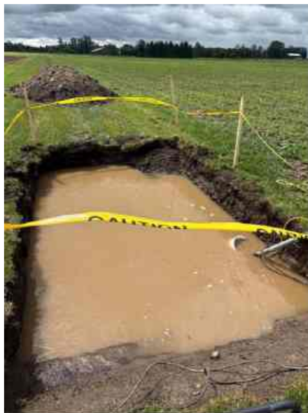
Photo 6. The Orthic Humic Gleysol soil pit was turned into an oversized bathtub after the rain. This soil pit was 110 cm deep, but the water table was only about 20 cm from the surface. Note the sump pump in the bottom right of the image.
